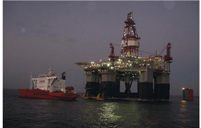
Choosing the right connectors is paramount when operating in harsh environments such as this sea-based oil rig. (Source: Jim Hatter via Wikipedia)
